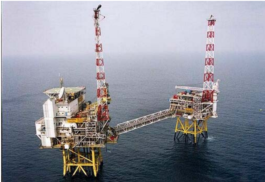
Fig. 0. The Draupner S and Draupner E platforms in the North Sea, Photo: Øyvind Hagen, Statoil.
